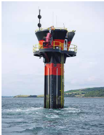
Figure 1. The world’s first commercial-scale tidal energy generator, SeaGen, in Strangford Lough, Northern Ireland. Reproduced under the Creative Commons Attribution-ShareAlike 2.0 licence.
