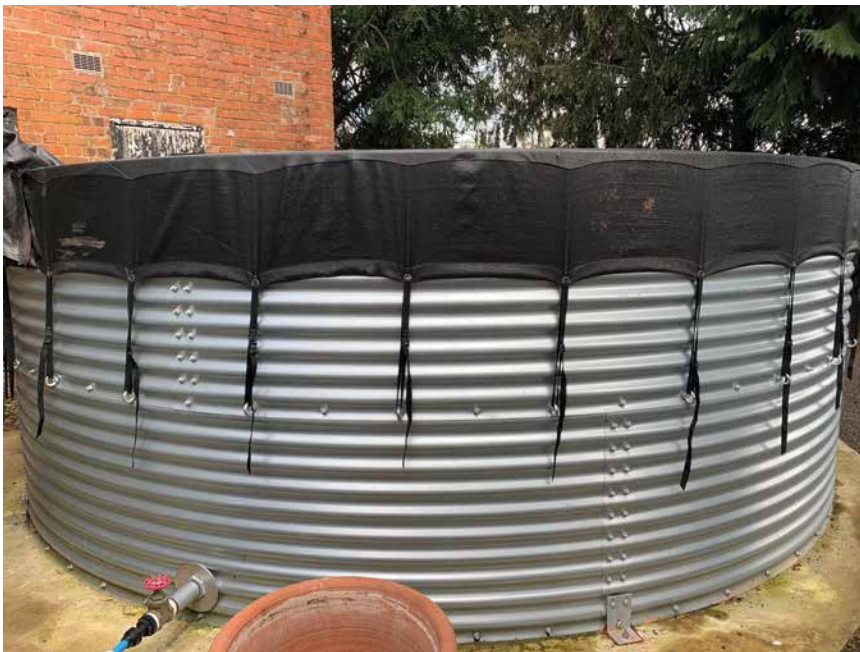
Figure 2. A rainwater harvesting tank at Powis Castle, Wales. Photo credit: National Trust.
