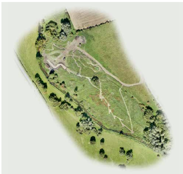
Figure 2. Aerial view of the site at the beginning of construction. Photo credit: Kev Morris.
